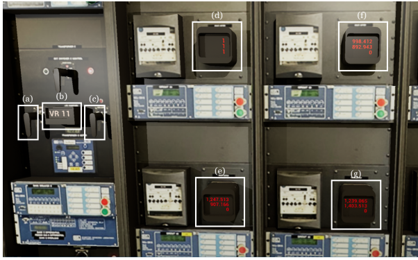
Fig. 7. Virtual substation HMI panels after phase C voltage at bus 671 has been restored to nominal range: (a) R2 breaker control switch, (b) Voltage regulator control, (c) R3 breaker control switch, (d) Bus 650 voltage meter, (e) Bus 650 phase A power meter, (f) Bus 650 phase B power meter, and (g) Bus 650 phase C power meter.
