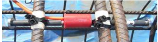
Fig. 3. Installed Strain Gauge on Pile Steel Cage
