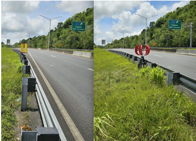
Figure 6: The Wind Turbines Installed at San Lorenzo Road
